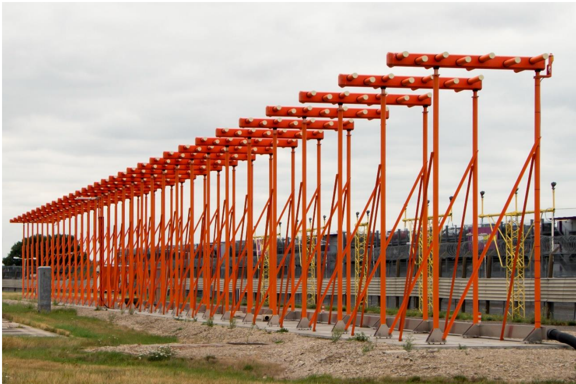
NORMARC Ultrawide Localizer with 32 elements
