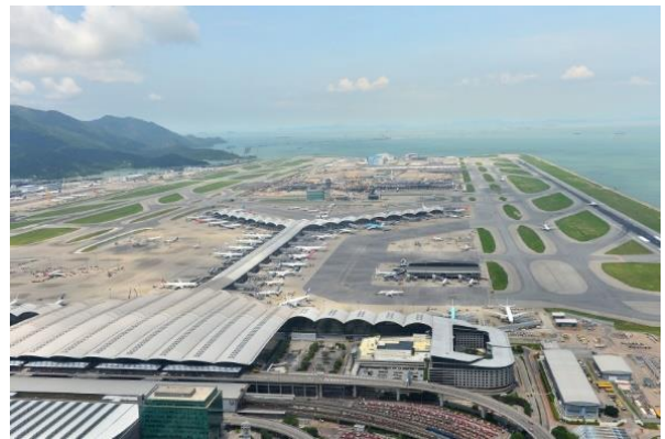
Hong Kong International Airport
